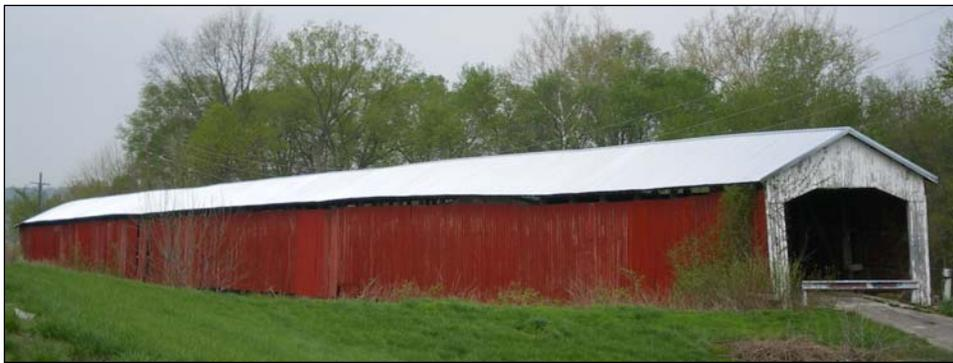
bridge has an overhang of 12 feet, and parts of it came from the Dixon quarry in nearby Fort Ritner. Having been bypassed in 1970, the bridge no longer supports traffic.<sup>7</sup>
